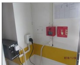
External photo(s) of the production unit(s) Fire alarm button and back-up battery.JPG
